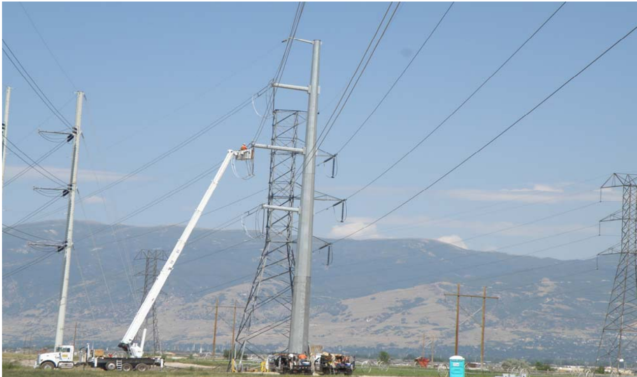
Angle Structure installation Ben Lomond to Terminal
