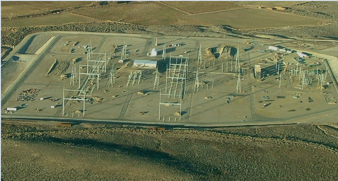
The Hemingway Substation under construction in Idaho. Three planned projects will connect here.
