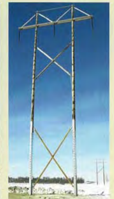
230kV H-Frame Structure Raised 20 feet
