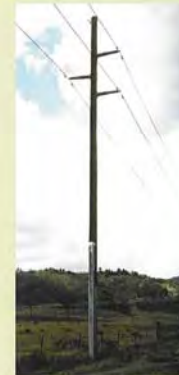
115kV Single Pole Structure Raised 10 feet
