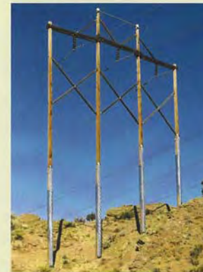
115kV Four-pole H-Frame Structure Raised 12 feet
