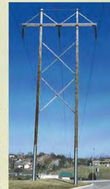
161kV H-Frame Structure Raised 5 feet
