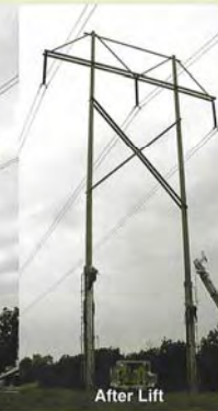
345kV H-Frame Structure Raised 15 feet
