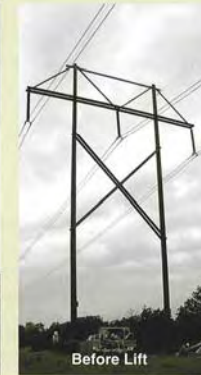
345kV H-Frame Structure Raised 15 feet
